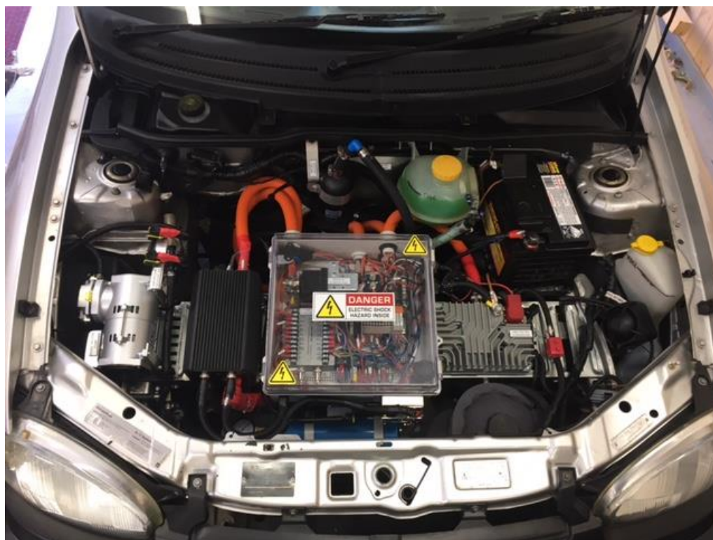
Top view of completed engine bay
